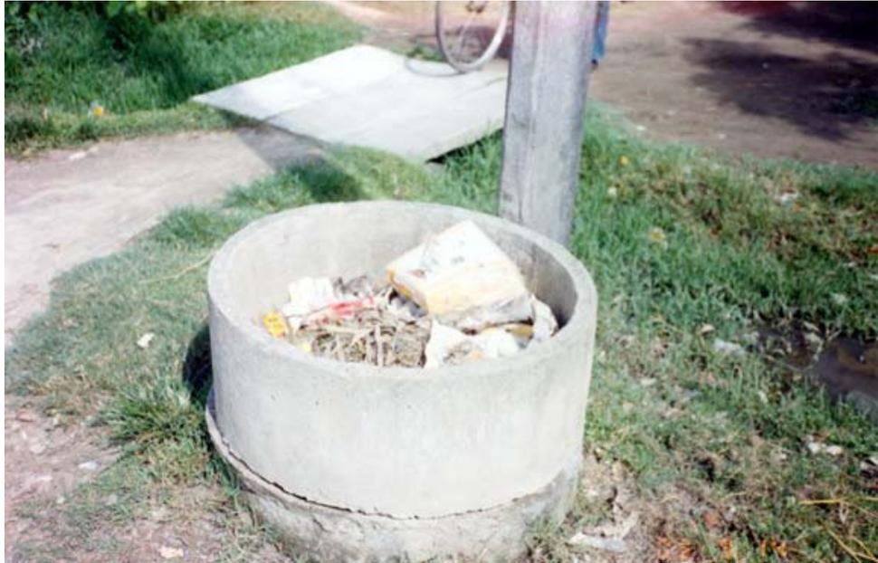
**Waste Container Made from Concrete Rings**
