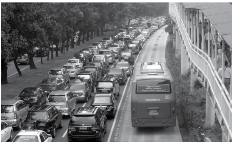
BRT system in Jakarta: right-of-way lane makes public transport competitive to car travel
