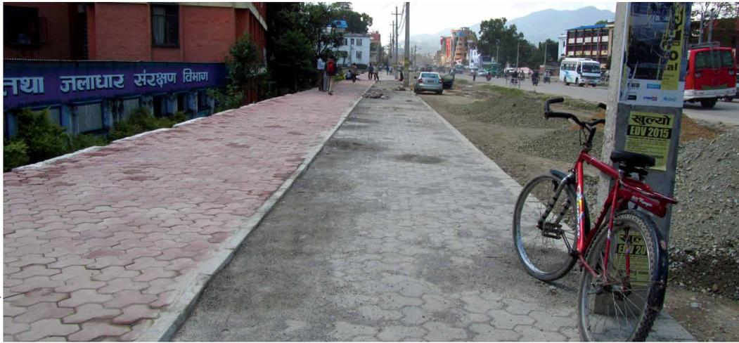
Fig. 11 Wrong paving materials used in newly constructed cycle track in Tinkune-Maitighar (Paver blocks and stone pavement should be avoided; smooth surface materials-asphalt or concrete preferred)
